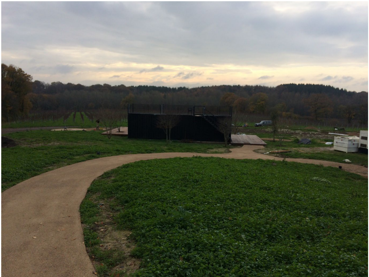
View of Garden Bar from Footpath
